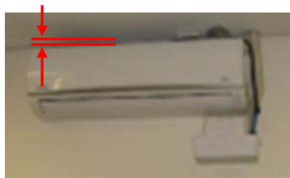
[Limited inlet airflow → temp. rise]
