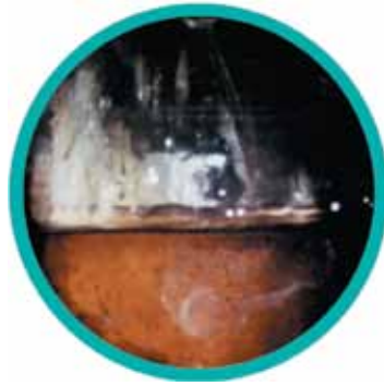
FIGURE 6-10: Liquid refrigerant enters compressor and settles to the bottom, below the oil.
