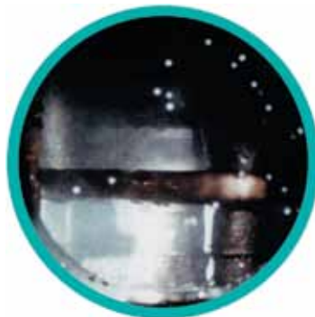
FIGURE 6-12: More than 60 seconds after start-up, oil level is well below normal operating levels - a condition that is an important factor in compressor bearing wear.
